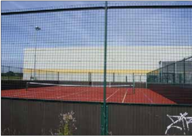
Figure 7.11 – Multiuse tennis courts at Rayleigh Leisure Centre
